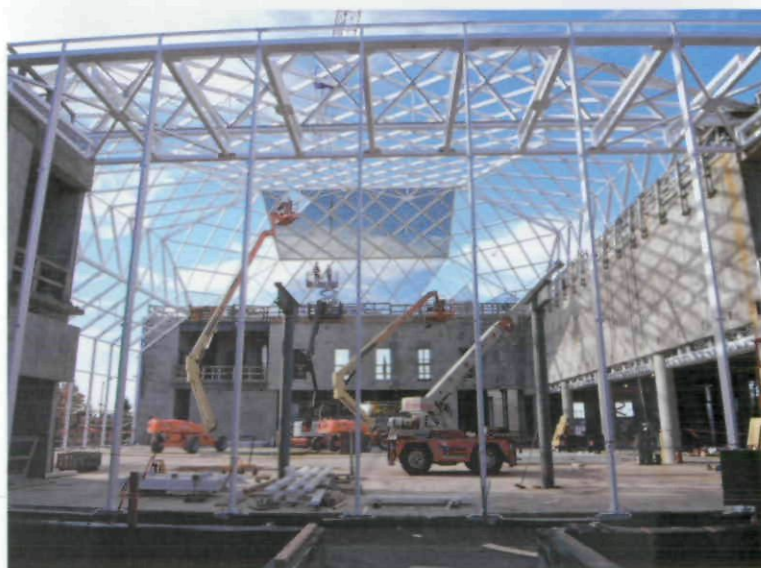
TOP DESCRIBED AS A "ROCK CRYSTAL," THREE LAYERS OF LOW-IRON GLASS SET ATOP A STRUCTURAL STEEL FRAME CONSTITUTE THE BUILDING'S MOST DYNAMIC ARCHITECTURAL FEATURE. ABOVE WORKERS MOVE TO INSTALL ONE OF THE 657 GLASS UNITS USED FOR THE ATRIUM'S ROOF.
